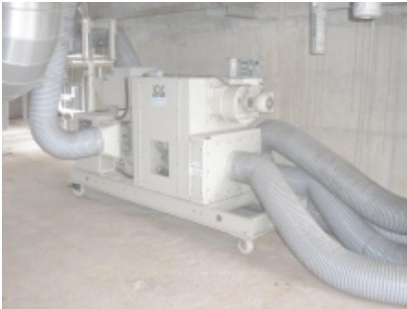
9, 10. Steam turbine has a separate dehumidifier (left) which is located external to the unit (right)
