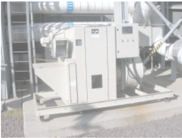
7, 8. Dehumidifier located outside the HRSG casing (left) works as illustrated at right
