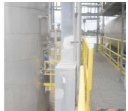
6. Duct balloon is simple to install through manhole accessible from catwalk
