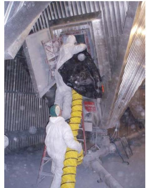
The duct balloon easily passes through the existing 27" x 21" man way during installation and weighs less than 25 lbs. Installation time takes minutes, not hours versus scaffolding.
