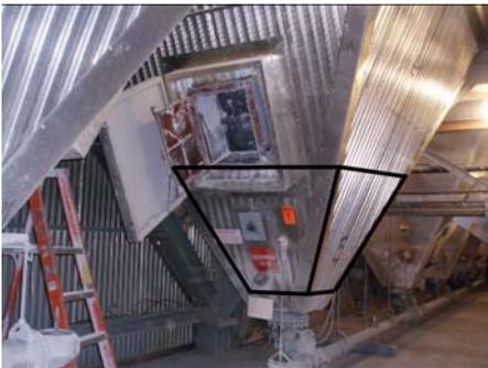
This installation is inside the bottom of an ash hopper on a precipitator. The inflatable platform will inflate so the top surface of the balloon is level with the bottom edge of the access door.
