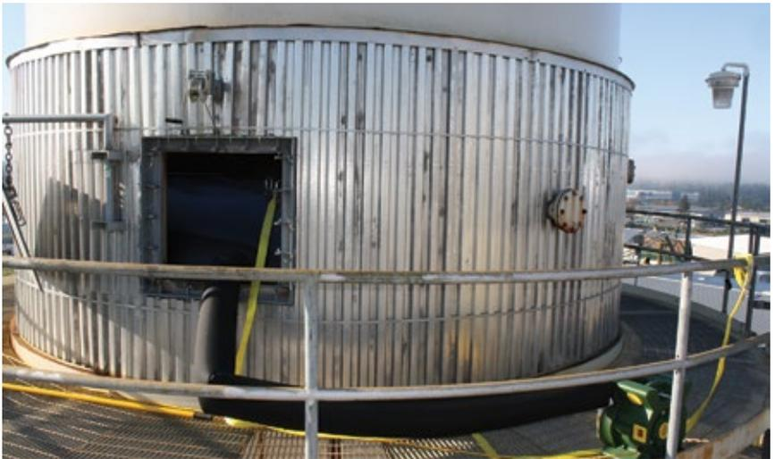
2. **Typical stack balloon slopes** toward the access for moisture drainage
